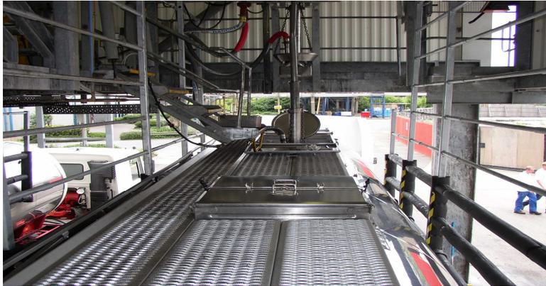
Alternatively, the required standard in top guarding can be achieved by raising the handrails provided on the road tanker. When the tanker is in position, sufficient clearance is required between the tanker and fixed steelwork structure to allow the handrails to be fully extended heightwise.
